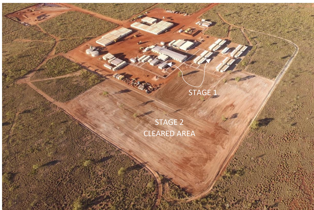
Figure 1 – Camp facility showing initial 60 rooms plus cleared areas for installation of remaining rooms.
