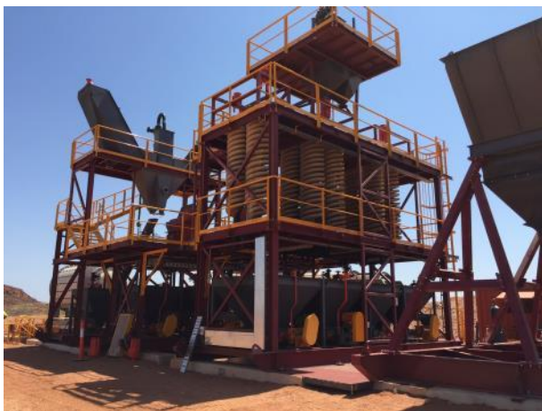
Tabba Tabba Processing Facility
