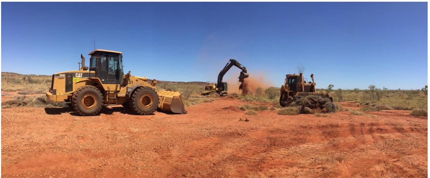
*Figure 1: Bulk earthworks underway at the Pilgangoora Lithium-Tantalum Project, Western Australia*
