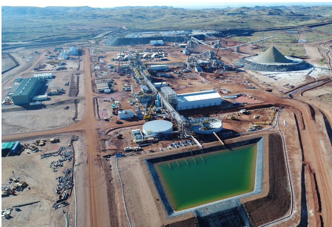
Figure 1 – Concentrator overview, with ore deliveries to the Run-of-Mine Stockpile in the background
