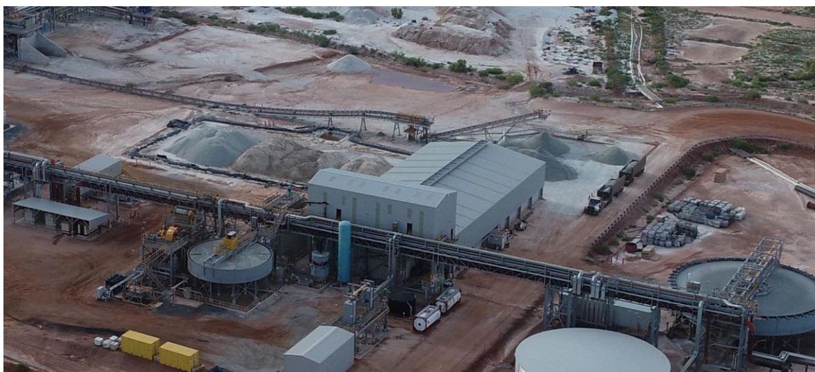
Final Product Shed and Stockyards, March 2020
