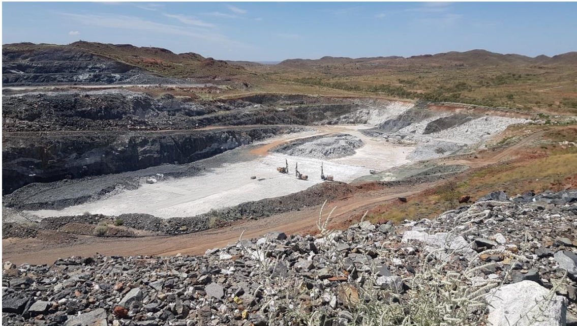
Central Pit – Drill and Blast March 2020
